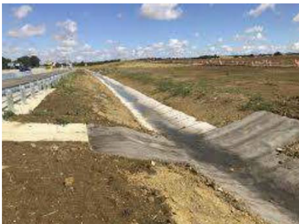
Figure 10: Typical Stormwater Concrete Lined & Grass Lines Channels
