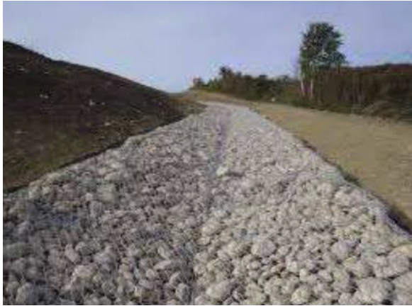
Figure 8: Typical Reno Mattresses for Steeper Portions of Stormwater Channels/Side Drains
