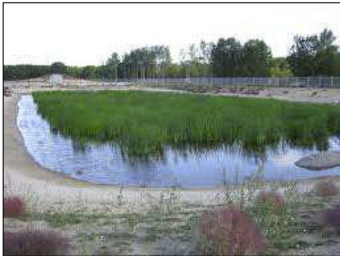
Figure 7: Typical Wetland Treatment Facility
