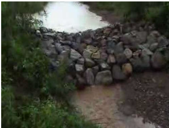
Figure 9: Typical Check Dam
