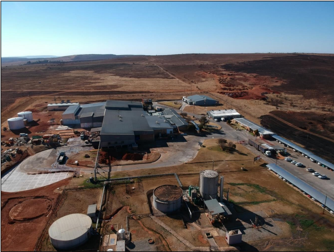
Figure 5: Processing plant prior to the expansion of the live bird receiving area, air-line chiller and gyro freezer
