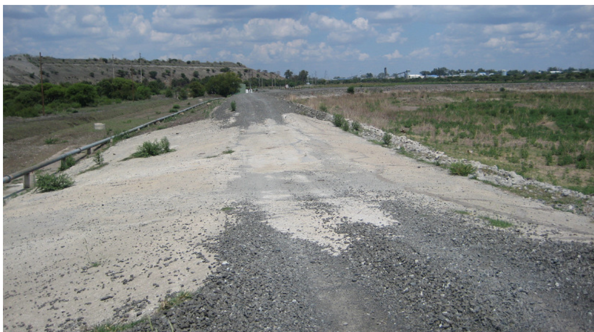
FIGURE 3-2: EMERGENCY SPILLWAY FROM UNION MINE RETURN WATER DAM (25 FEBRUARY 2016)
