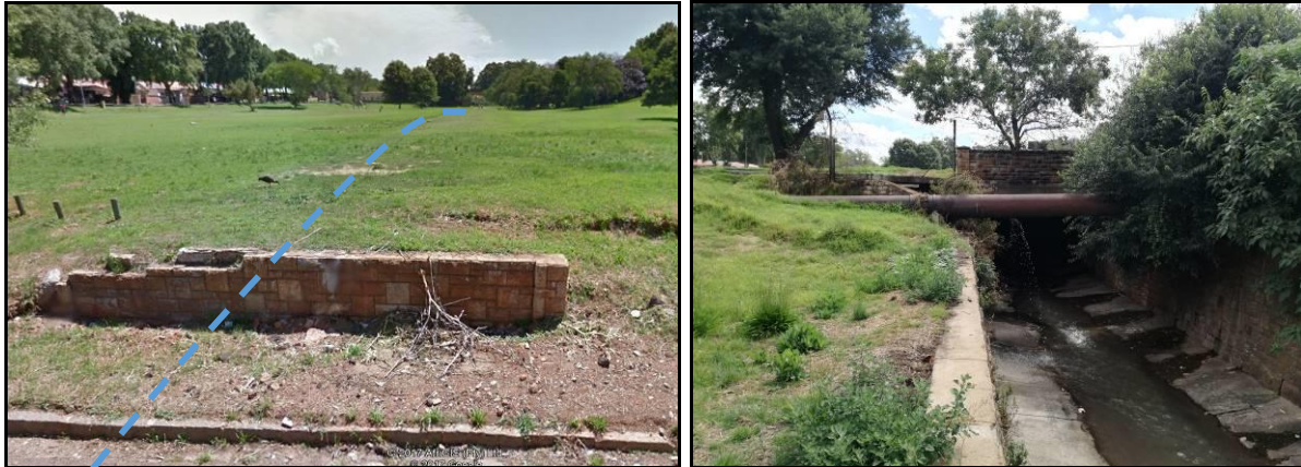
Figure 4: Left: The area west of 6 th Street where the canal is underground (blue line), before it daylights to the east of 6 th Street. Right: The canal daylights east of 6 th Street, south to the clinic property (located to the right in this photograph).
