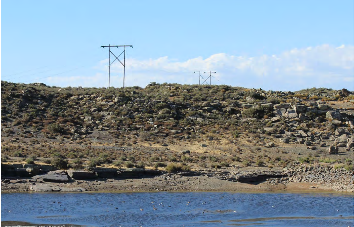
Figure 1-23 View north-west from SVP005 next to the Theronrus farmstead. An existing 132 kV power line exposed above the ridge - the power line follows along most of this road.
