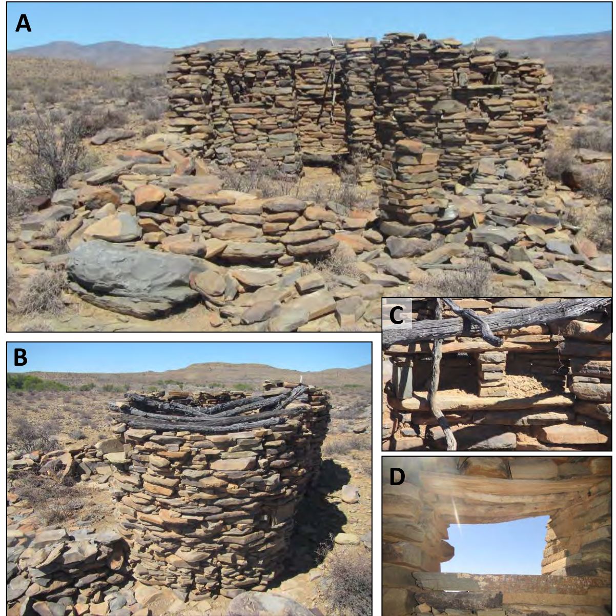
Figure 29: Plan of the stone-walled house at waypoint 500 with (A) a view towards the west of the entrance, (B) a view towards the south of the northern lobe showing remaining roof 'beams', (C) a view of the high 'muurkas' in the western lobe and (D) a view of the east-facing window with wooden planks and sticks in the southern lobe. Not to scale but approximate measurements are indicated.
