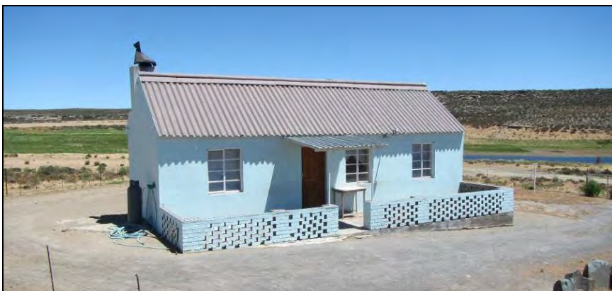
Figure 38: The small cottage close to the dam at waypoint 506.
