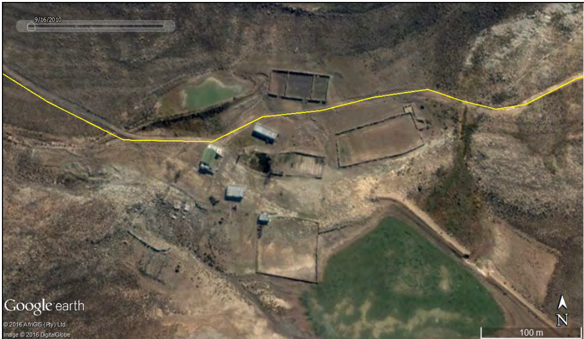
Figure 40: Aerial view of the Gunstfontein farm complex with the proposed power line route along the road in yellow.
