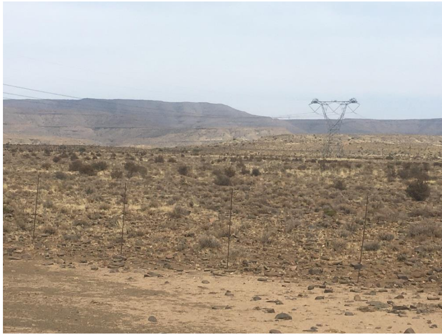
View of the existing Eskom power lines south of the proposed 400 kV power line from Portion 7 of Farm Hamelkraal 16 (Source: Shawn Johnston).
