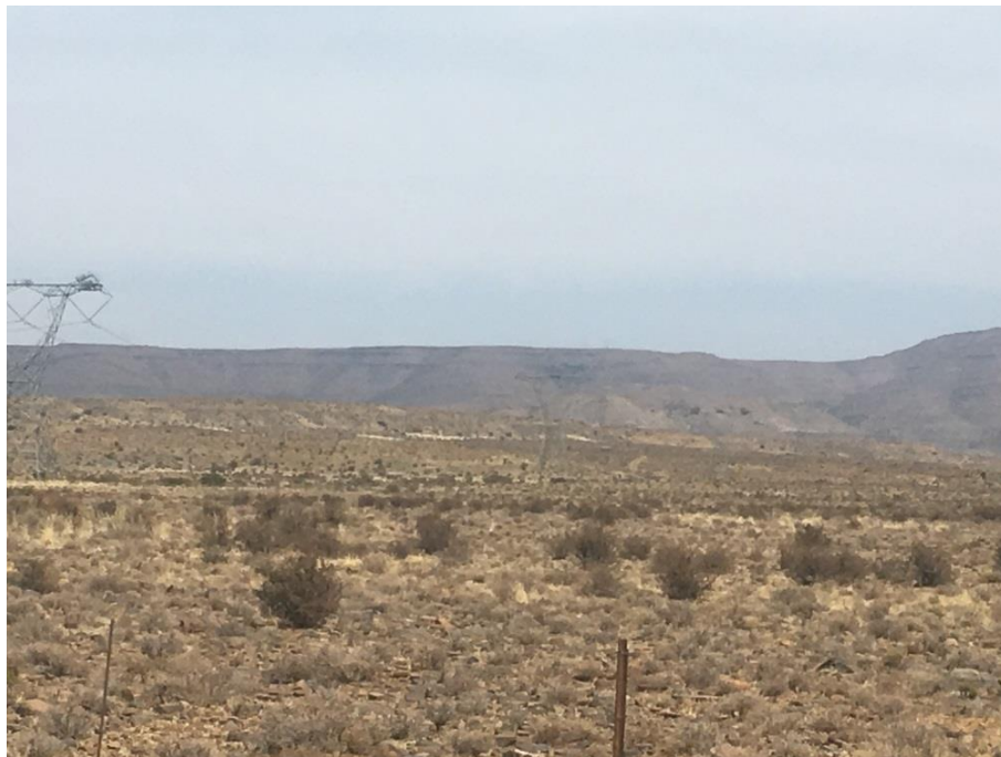
View of the existing Eskom power lines south of the proposed 400 kV power line from Portion 7 of Farm Hamelkraal 16 (Source: Shawn Johnston).
