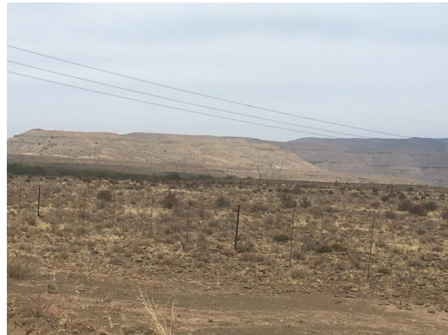
View of the existing Eskom power lines south of the proposed 400 kV power line from Portion 7 of Farm Hamelkraal 16 (Source: Shawn Johnston).
