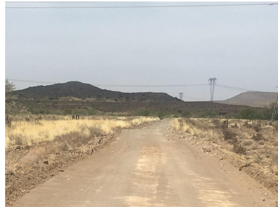
View of the existing Eskom power lines south of the proposed 400 kV power line from Portion 7 of Farm Hamelkraal 16 (Source: Shawn Johnston).
