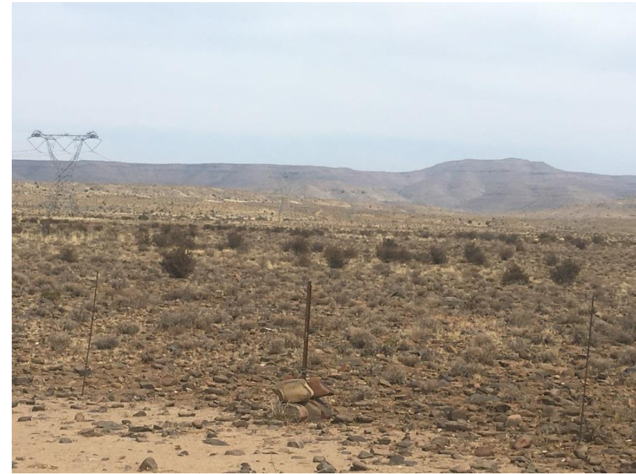
View of the existing Eskom power lines south of the proposed 400 kV power line from Portion 7 of Farm Hamelkraal 16 (Source: Shawn Johnston).
