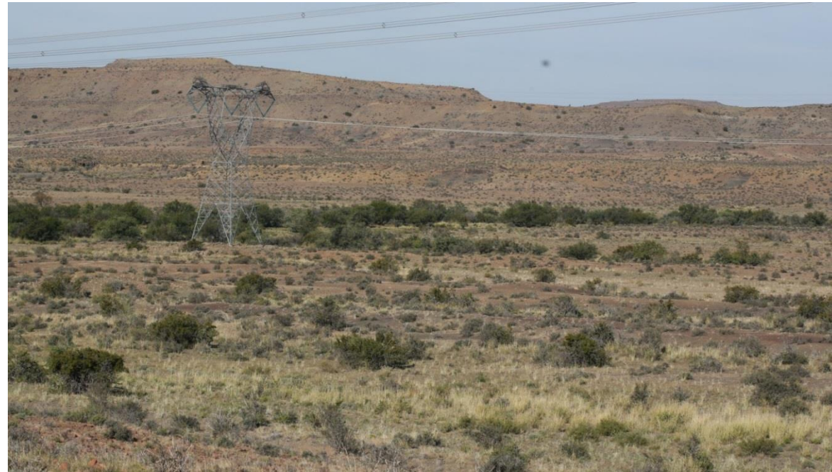
Towards the Eskom 400 kV power line where the current planned 400kV lines would link into the existing line (Source: Terrestrial Ecology Impact Assessment, Appendix D.1 of the BA Report).
