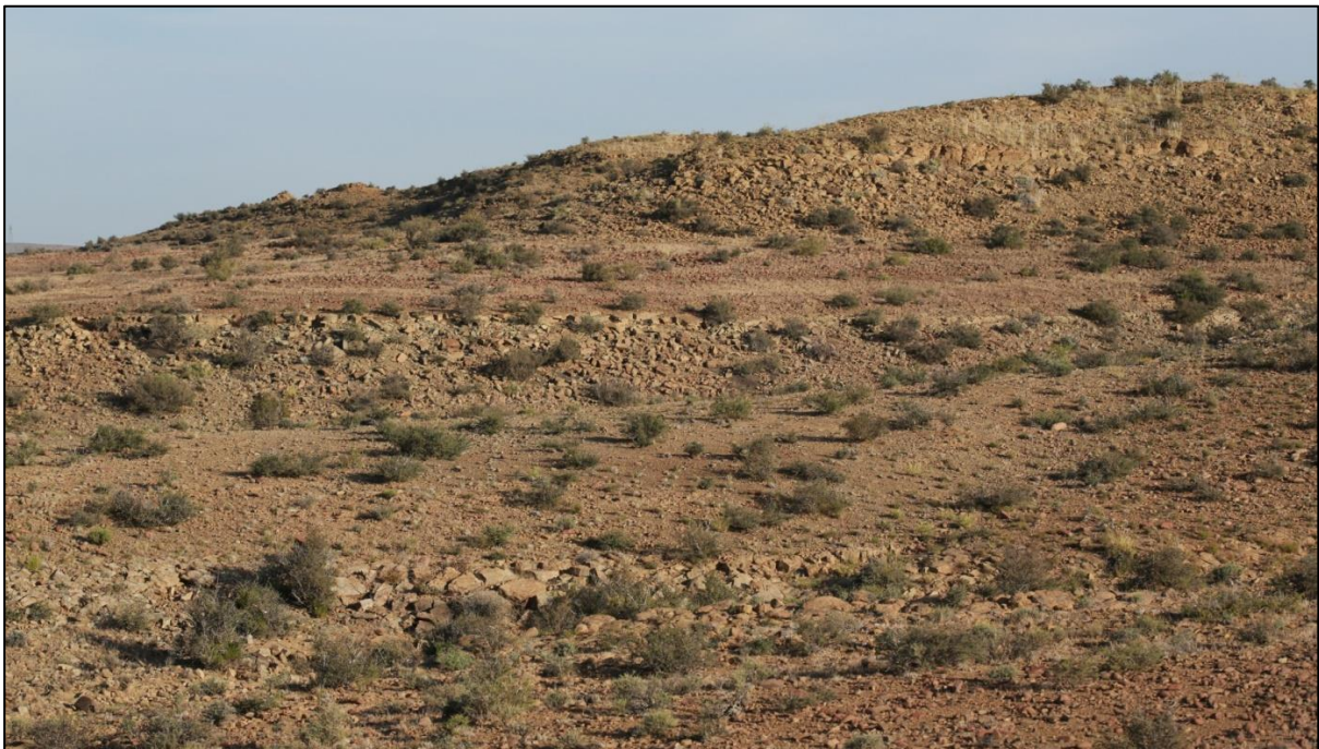
Figure 5. Looking south over the substation site from near the northern boundary of the site.
