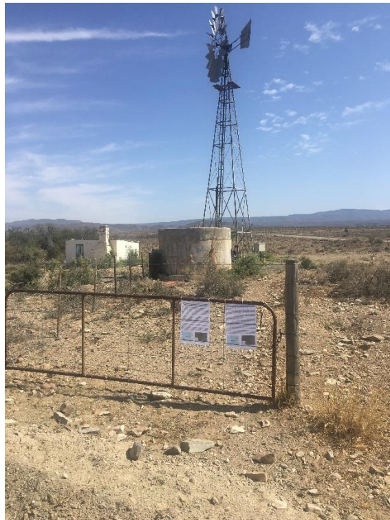
Site Notice Board 4 (English and Afrikaans) placed along the proposed 132 kV Power Line Route on Portion 6 of Farm Hamelkraal 16.
