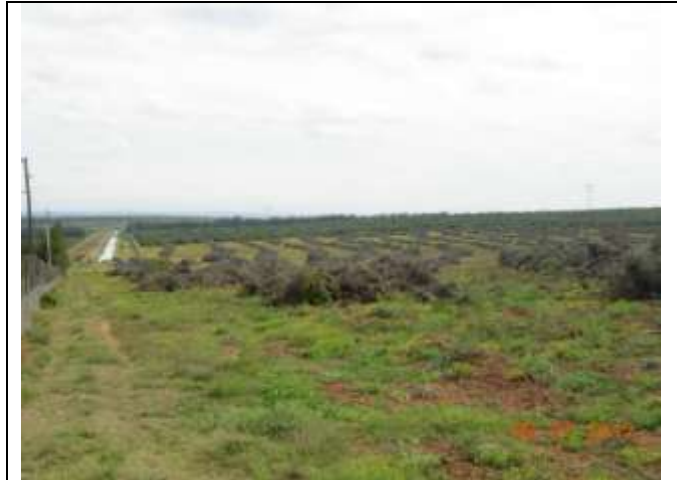
Photo 2.1 Vegetation cleared on site and stockpiled in rows.
