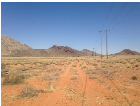
Figure 7: Existing powerline and single track road
