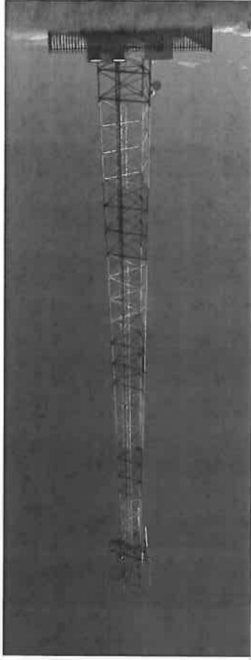
TYPICAL LATTICE MAST PAINTED RED & WHITE
