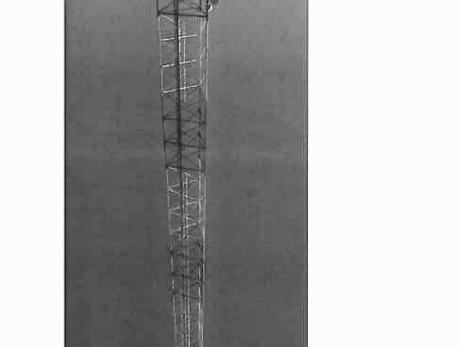
TYPICAL LATTICE MAST PAINTED RED & WHITE
