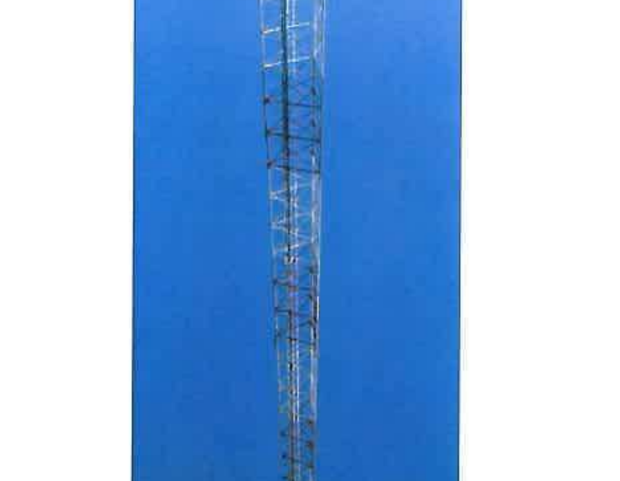
TYPICAL LATTICE MAST PAINTED RED & WHITE
