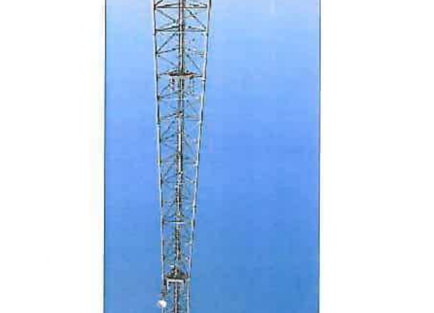
TYPICAL 3-LEGGED GALVANISED (UNPAINTED) LATTICE MAST
