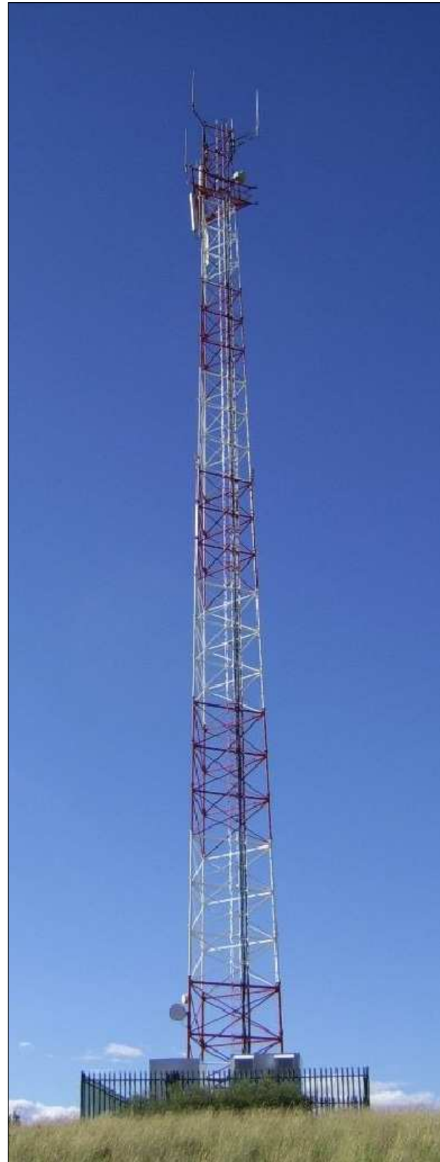
TYPICAL LATTICE MAST (PAINTED RED & WHITE)
