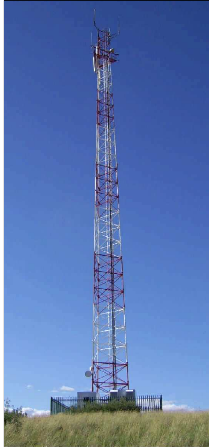
TYPICAL 3 LEGGED LATTICE MAST (PAINTED RED AND WHITE)
