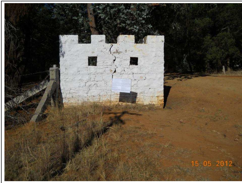
Site Notice 2 affixed to temporary stand next to old building
