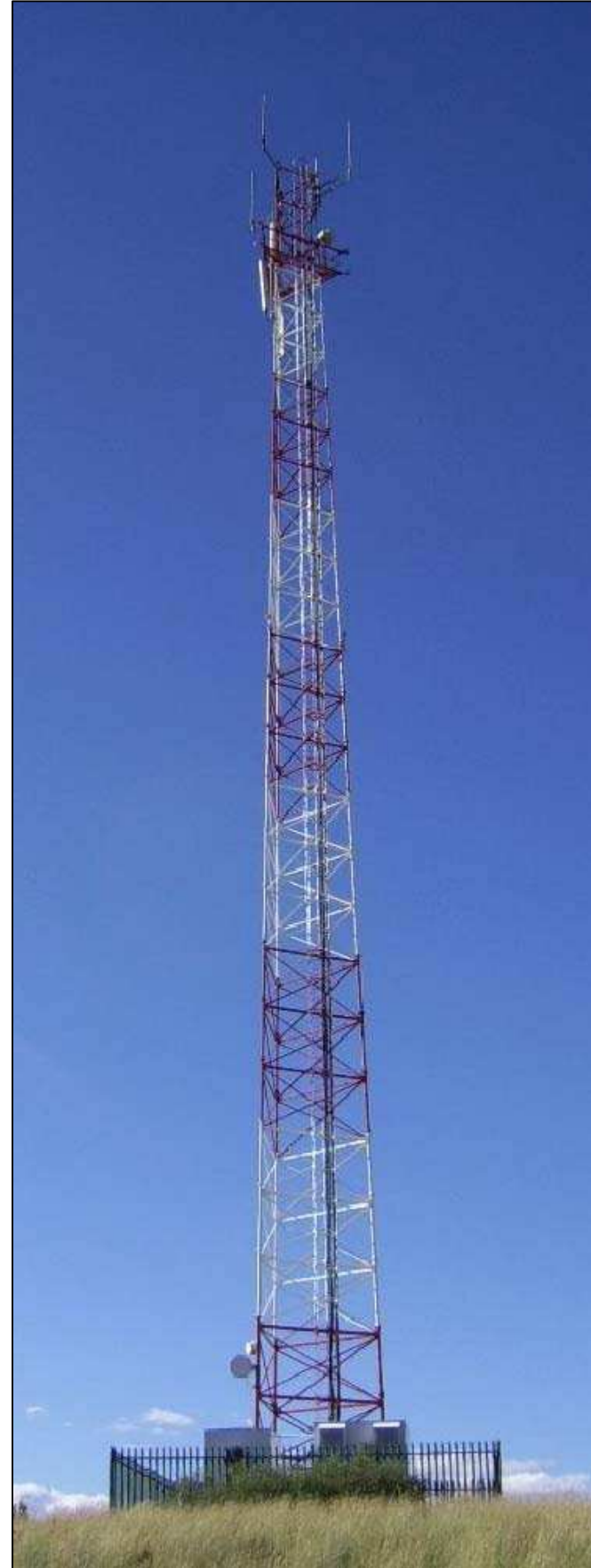
TYPICAL LATTICE MAST (PAINTED RED & WHITE)
