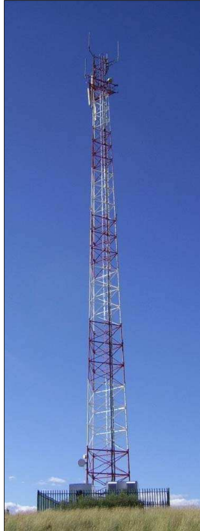
TYPICAL LATTICE MAST (PAINTED RED & WHITE)
