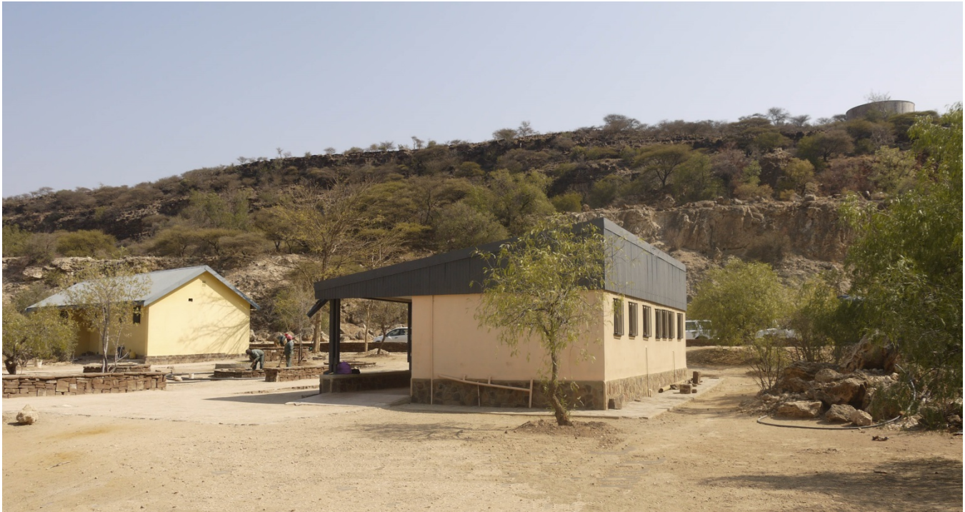
Fig 13: existing abluition block
