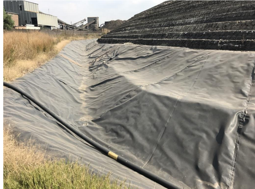
Leachate and storm water channeling around perimeter of Fe-Cr WDF
