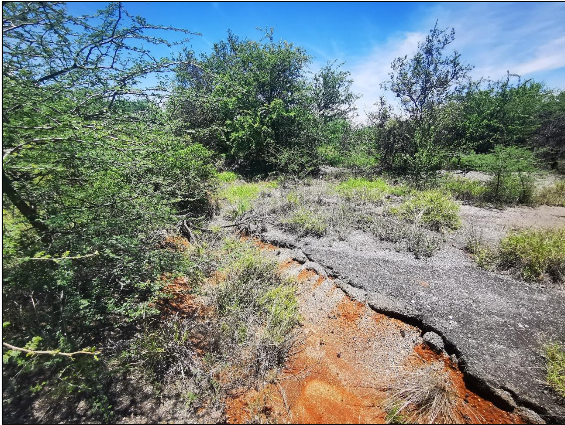
Figure 5-7 Illustration of concrete within the bed of the tributary
