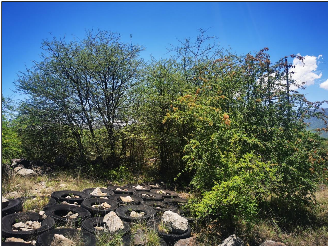
Figure 5-8 Illustration of tyres used for erosion control
