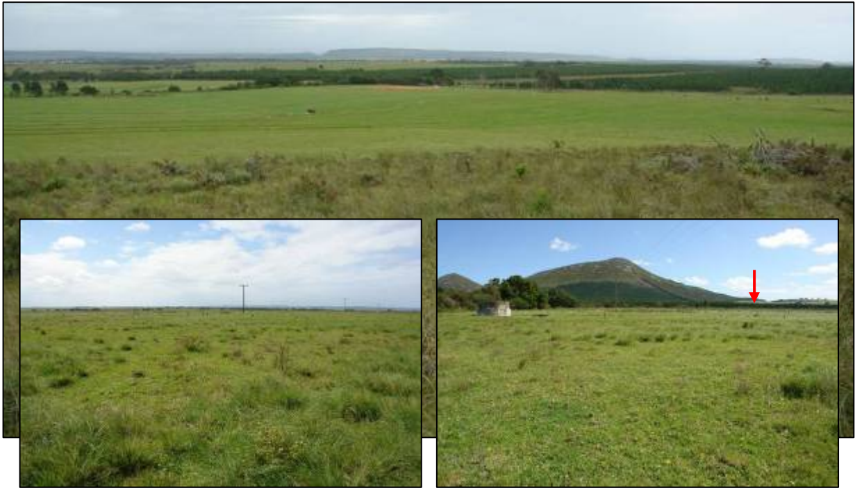
Figure 1. General views of the TCWEF landscape from where the powerline will be constructed (main image and left insert) towards the N2 (left insert) en route to the Dieprivier substation (right insert). The N2 runs at the foot of the hill and the red arrow marks the area where the route passes over the low foreland hills.
