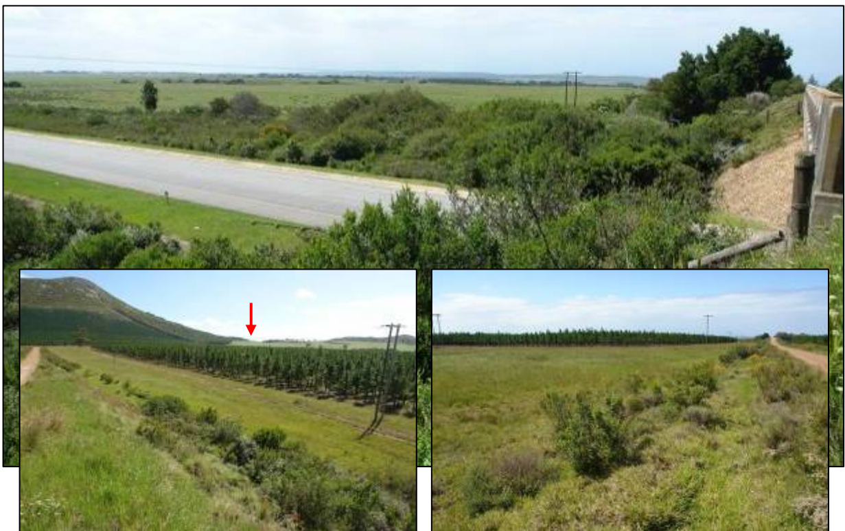
Figure 2. Views of the powerline route from the TCWEF substation towards the N2 (main image) and from the N2 towards the R102 and the low foreland hills (inserts). The red arrow marks the area where the route passes over the low foreland hills.
