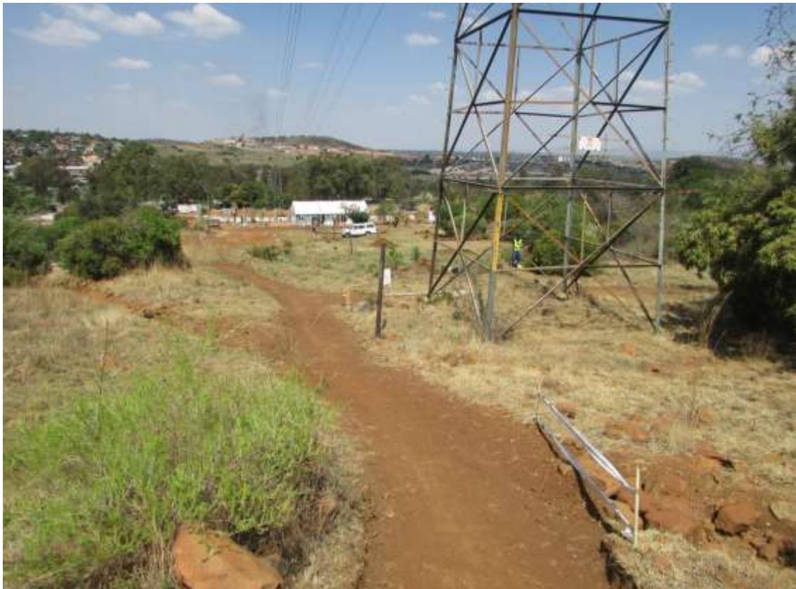
Figure 18: The impacts of the Eskom Powerlines and pylons, as well as hiking trails on the site is evident here.
