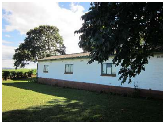
Fig 30: Edge from the access road
