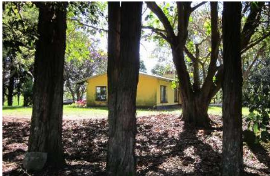
Fig 27: Estate management house 2
