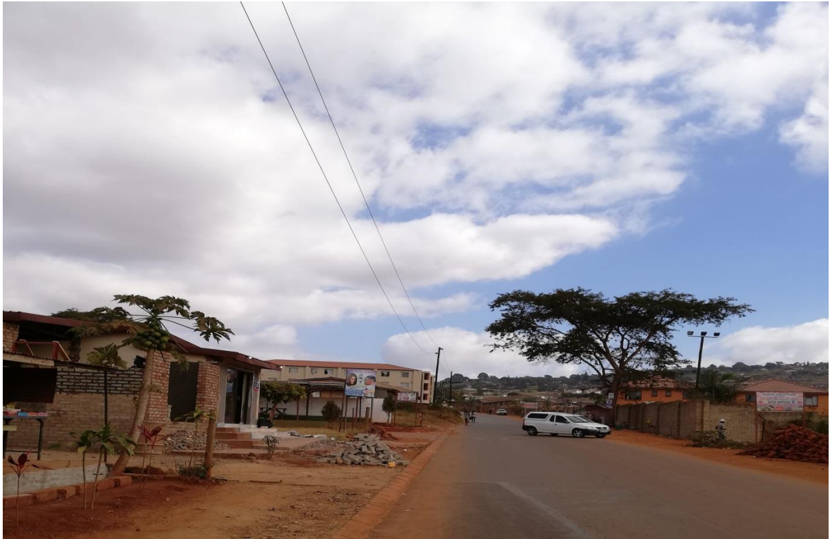
Picture showing the existing powerlines, tarred road and houses
