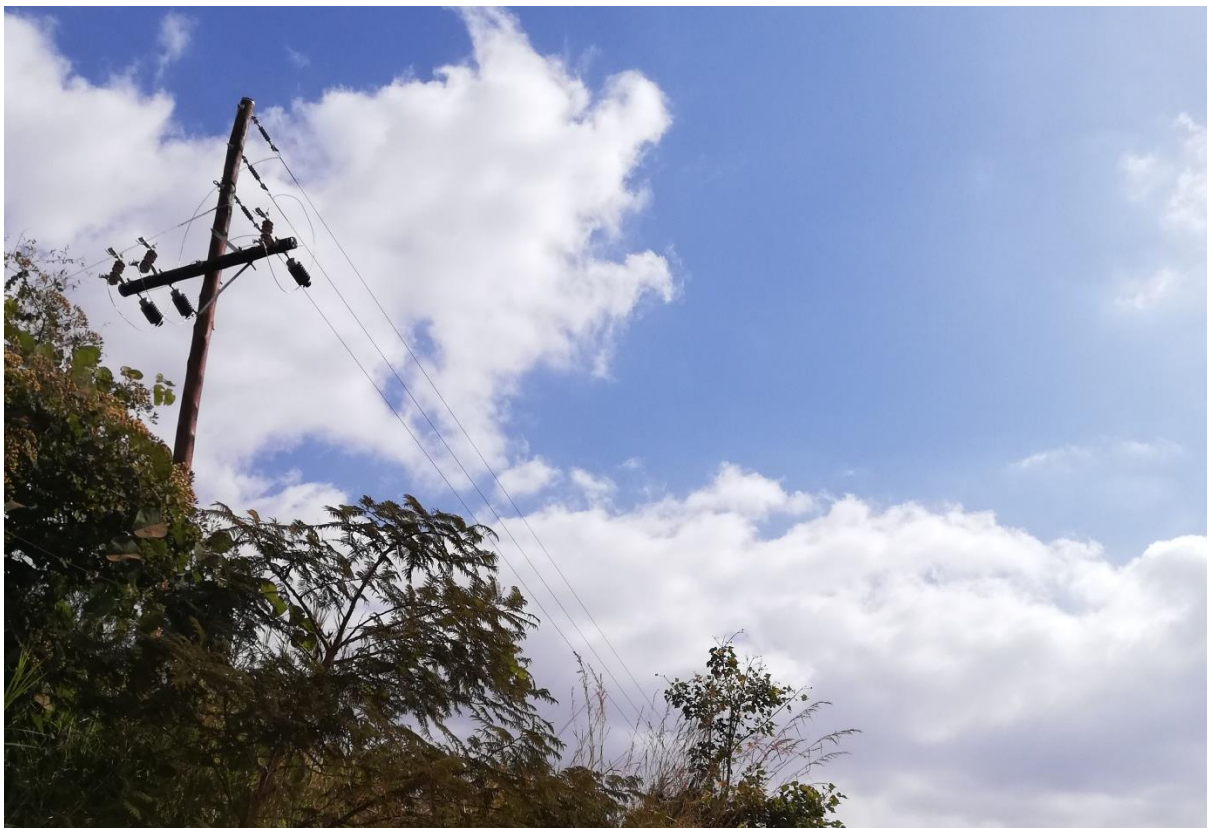
Picture showing where the powerline is going to be connected
