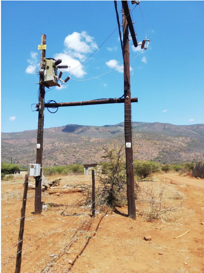
Figure 3 The T- Off Pole
