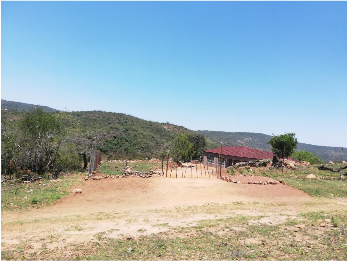
Figure 6 The power line crosses the small dirt road to supply the customer's yard
