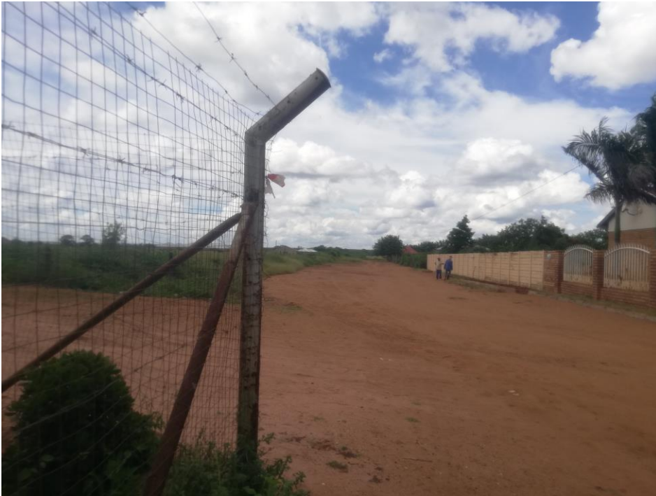
Figure 5 One of the pole positions on site
