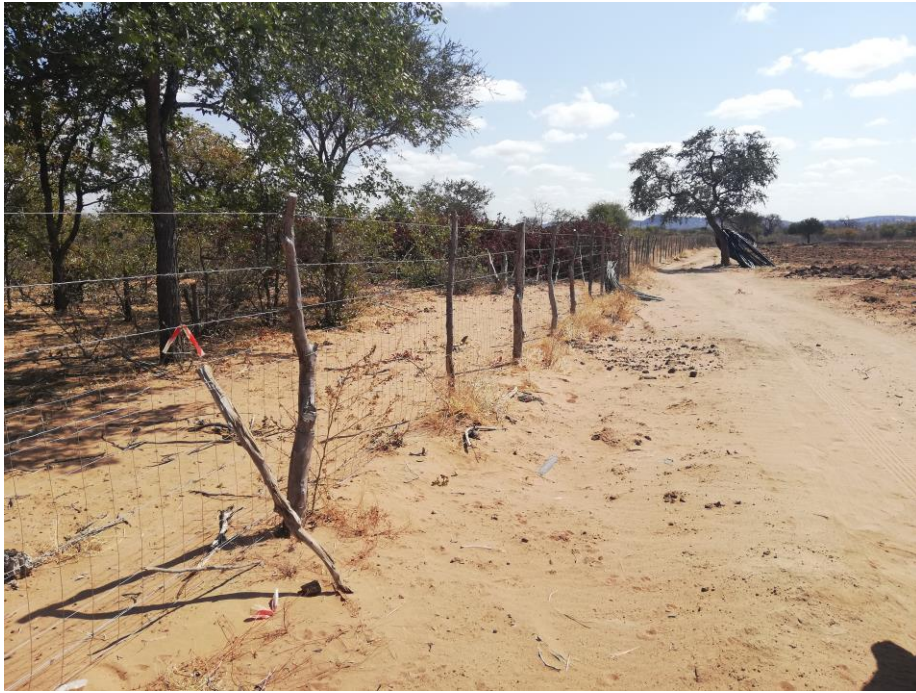
Figure 9 Transformer position peg. The line runs along the boundary fence
