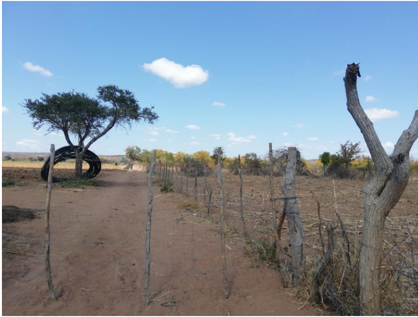
Figure 7 The power line runs along the fence
