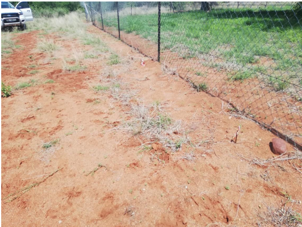
Figure 5 Point of Supply
