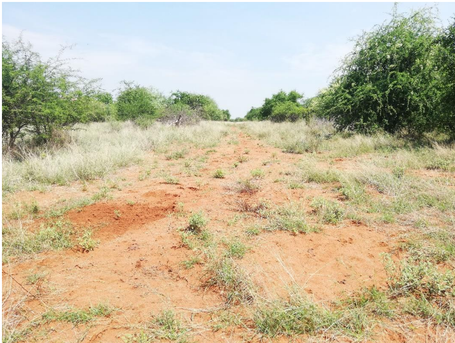
Figure 2 The corridor of the power line
