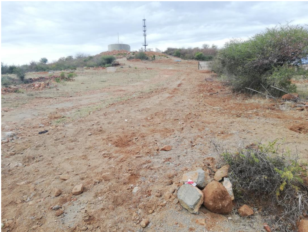
Figure 6 Pole position and telecoms tower to be supplied
