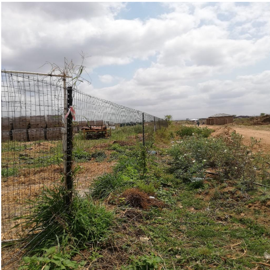
Figure 4 One of the pole pegs
