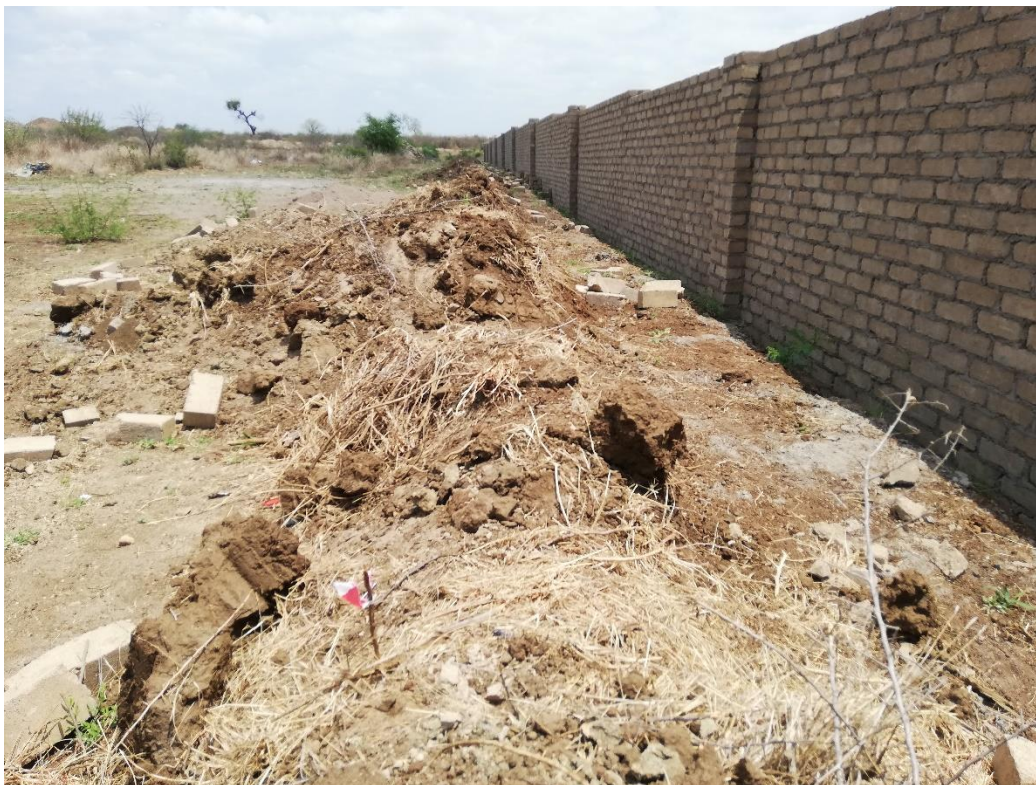
Figure 6 Transformer position within the customer's yard
