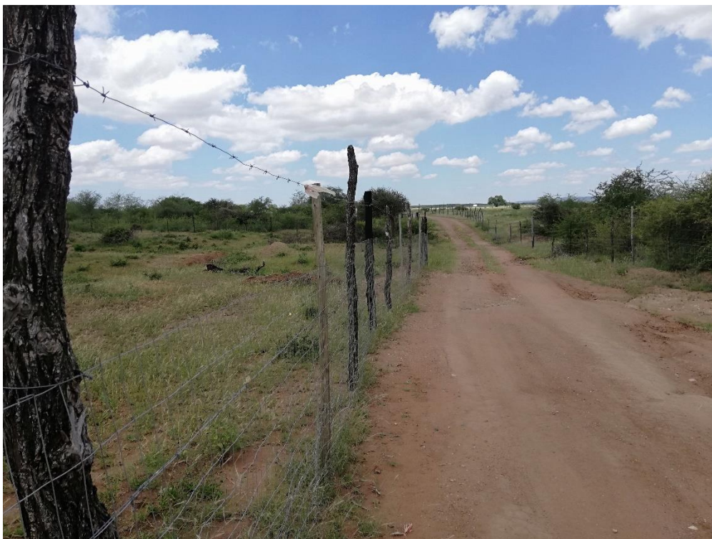
Figure 6 The power line runs parallel to the boundary fence
