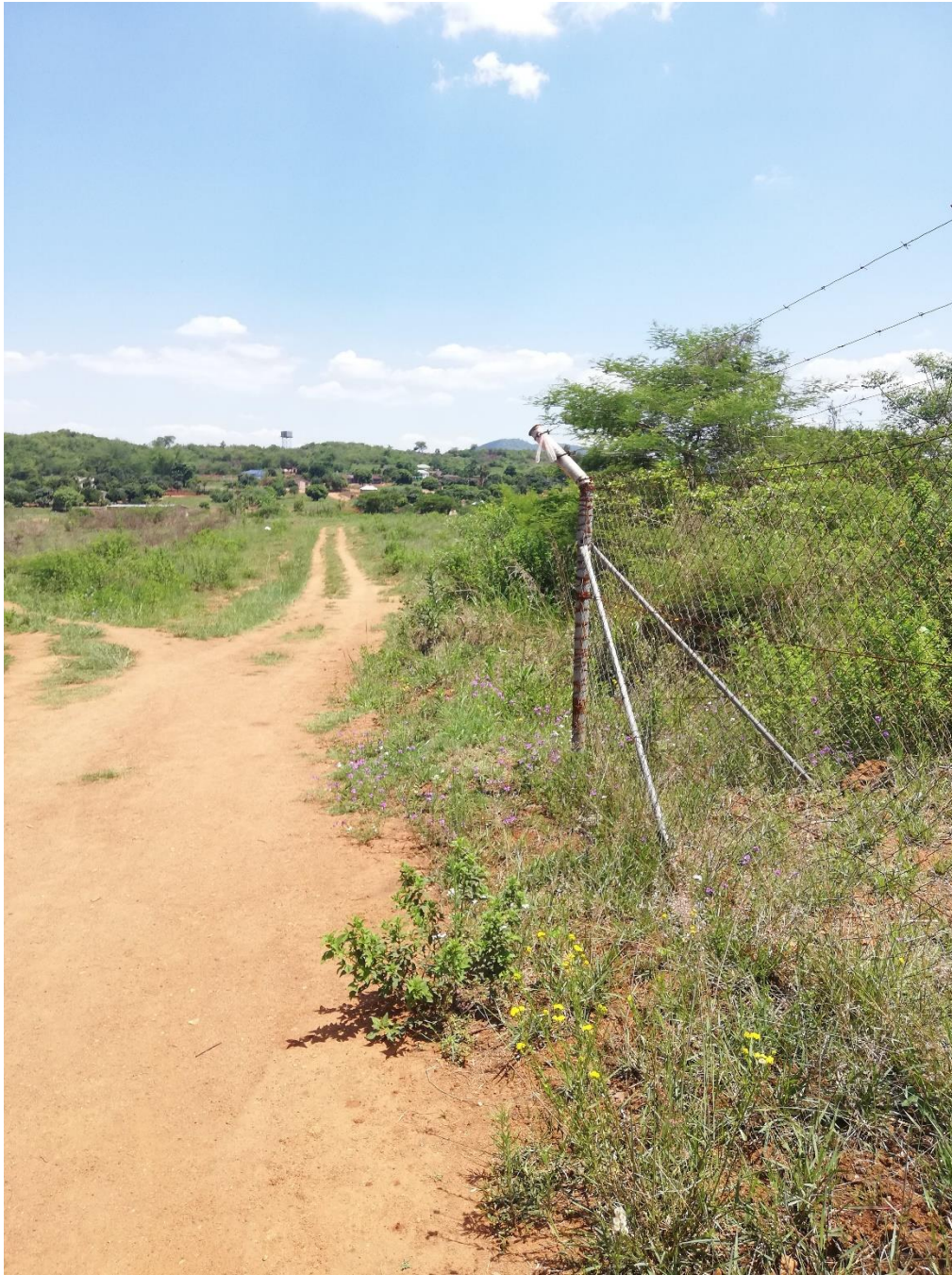
Figure 6 The power line continues along the dirt road
