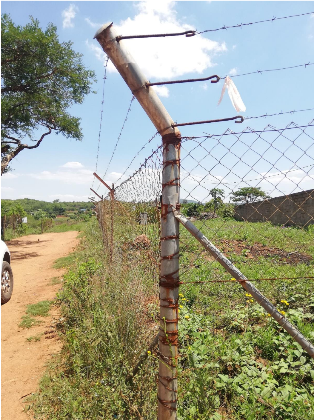
Figure 5 The power line runs parallel to the fence
