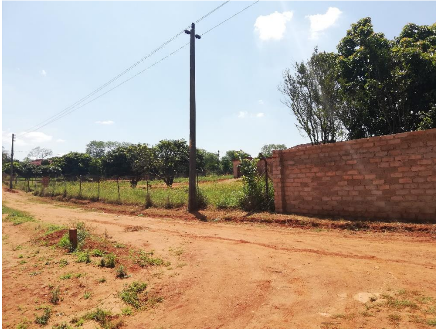
Figure 1 The existing power line on site
