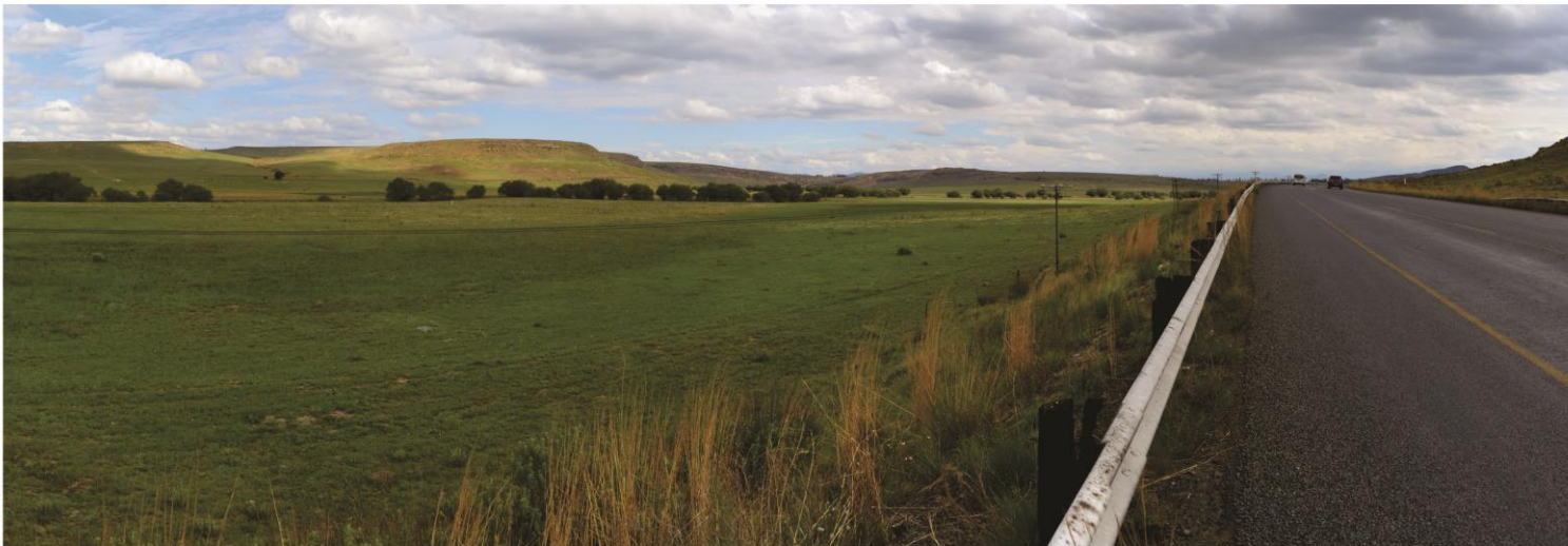
Photo 8: Plug-in (323 E & 324 F) located along Th R74, Harrismith
