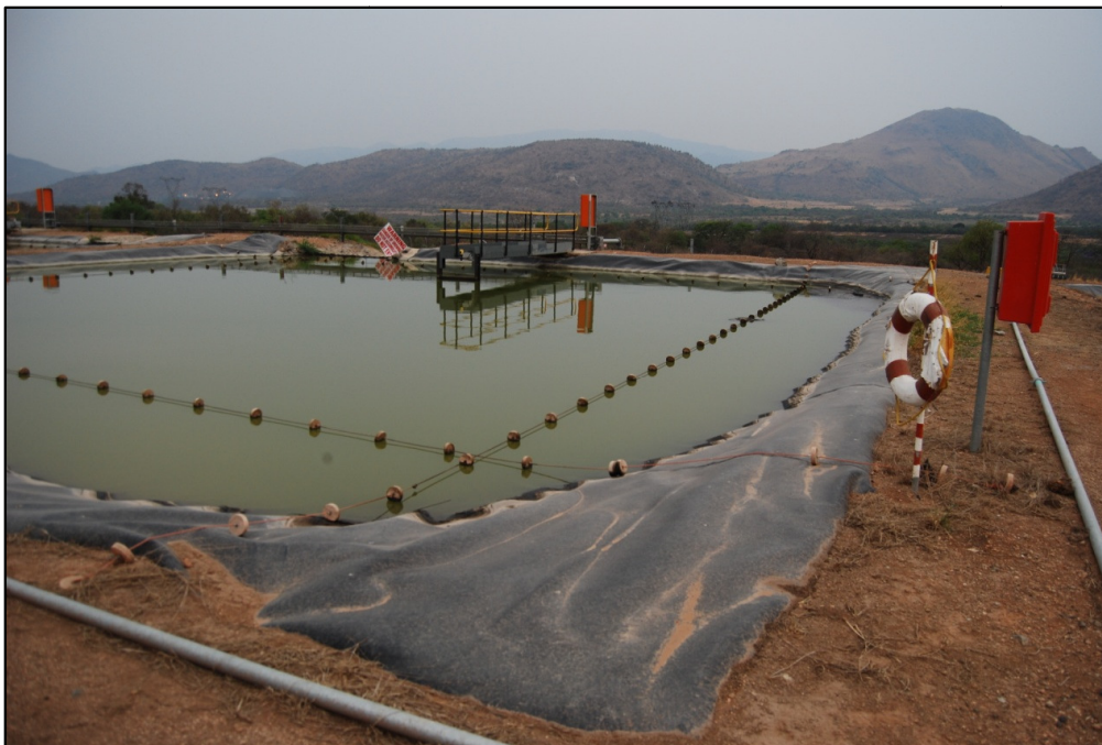
Photo 3.4 Existing PCD at the North Decline, currently operational
