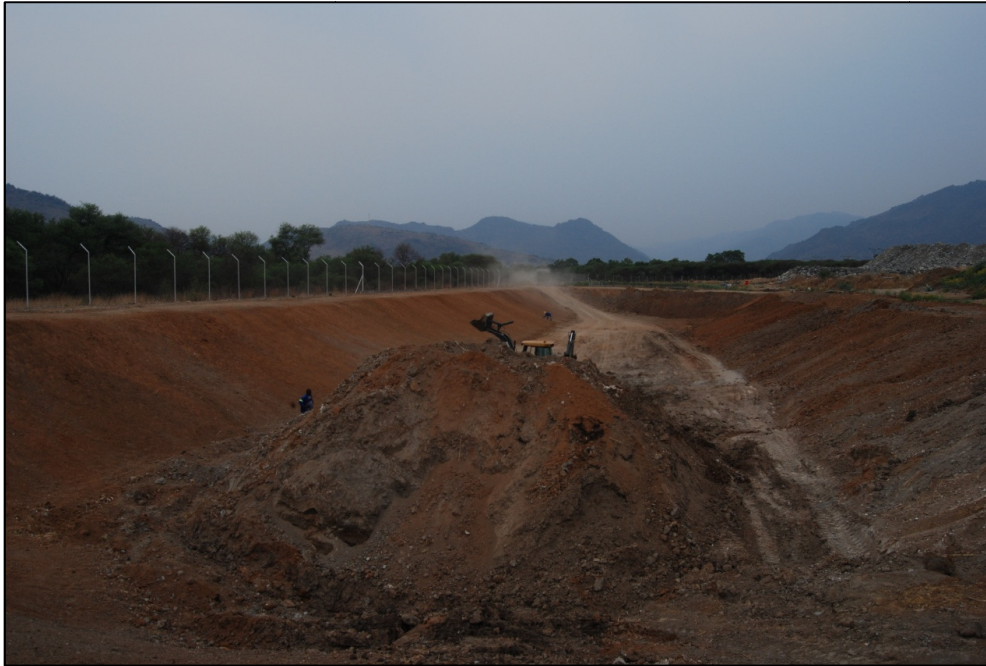
Photo 3.1 New PCD at the Main Decline, during construction Phase
