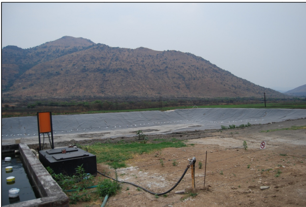
Photo 3.2 New PCD at the Plant, Prior to operation
