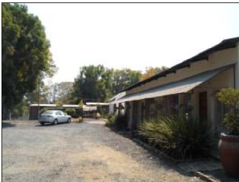
Photo 2.5 Buildings present on the New TSF site
