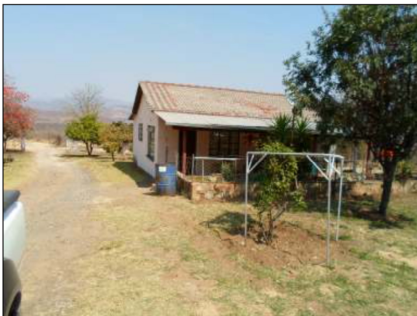
Photo 2.1 Buildings present on the New TSF site
