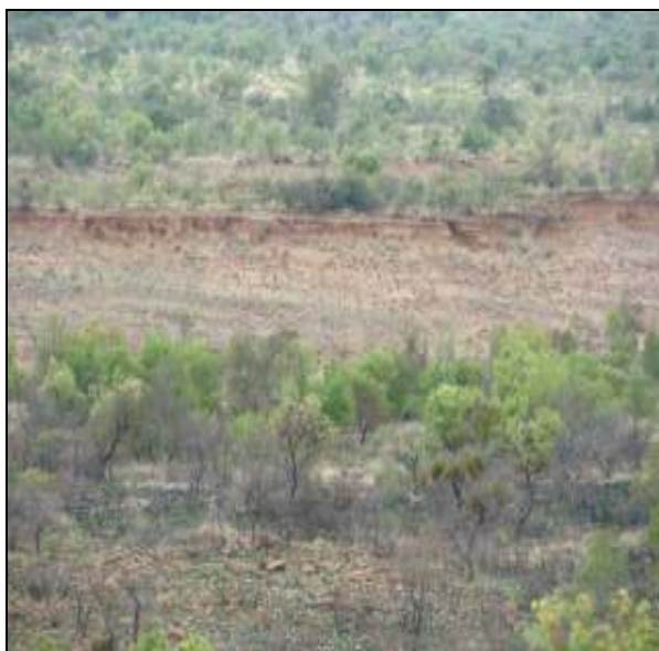
Photo 5.5 One of the erosion dongas within project area
