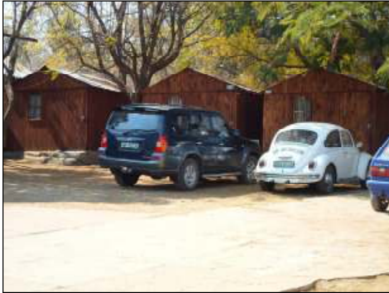
Photo 2.3 Buildings present on the New TSF site
