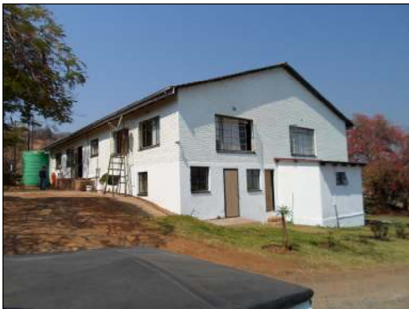
Photo 2.2 Buildings present on the New TSF site
