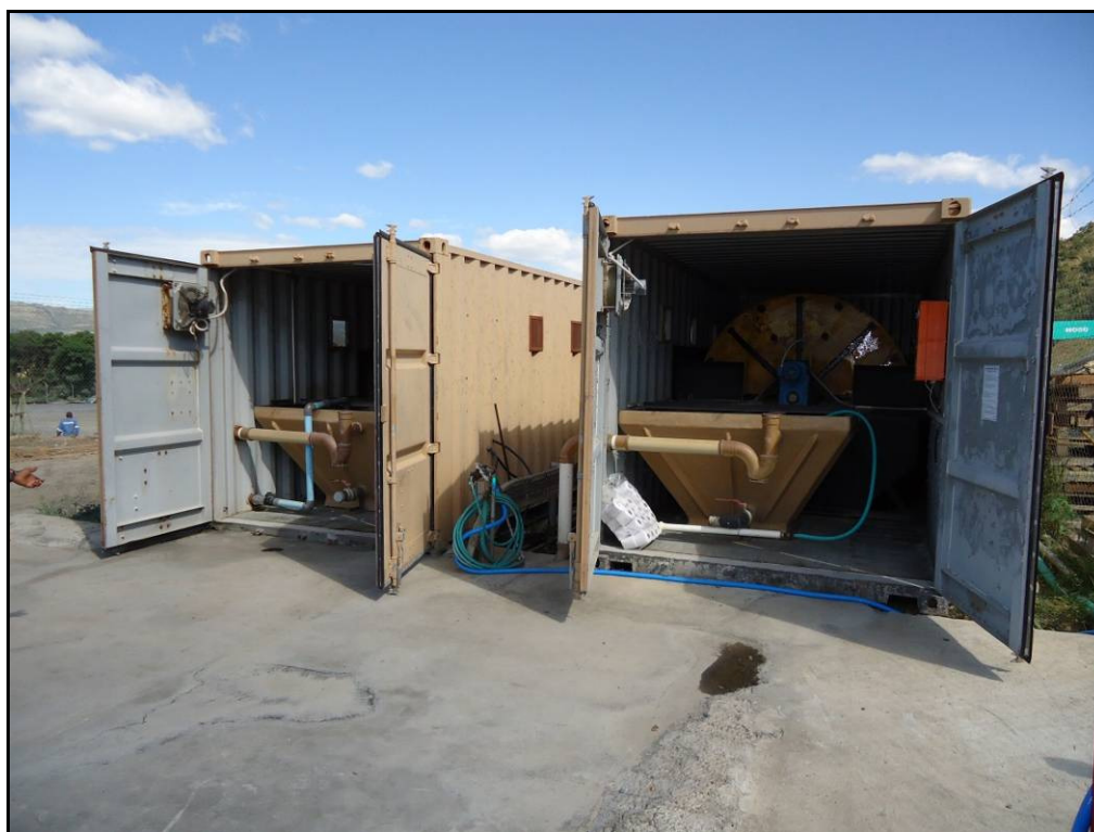
Photo 4.1 Sewage Package Plant Layout
