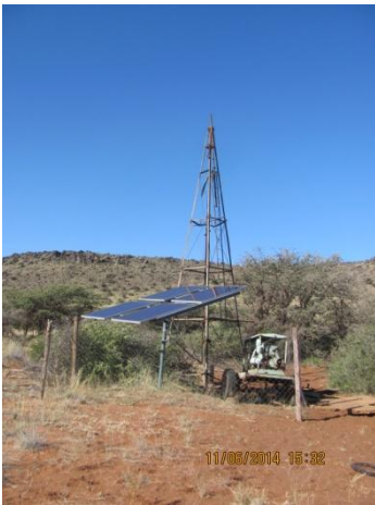
Figure 18: Solar pump and borehole.
