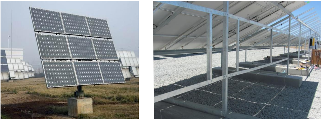
Figure 6: Examples single axis & fixed solar cast foundations.
