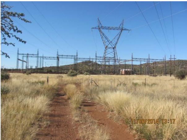
Figure 13: Steel-lattice powerline extending from east, across 4/436.
