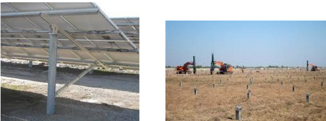
Figure 7: Typical rammed or screwed method of installation.
