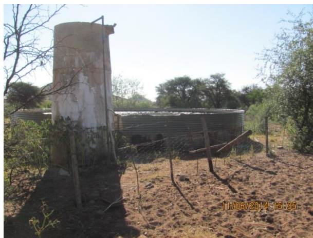
Figure 17: One of two water reservoirs connected to borehole / solar pump.
