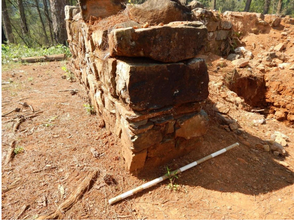
Fig. 3: The entrance to the burial site in the western wall. The wall is approximately 500mm wide.
