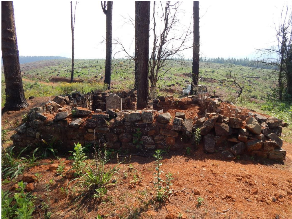
Fig. 6: The eastern wall has been damaged, mostly at the top. It is not clear if the damage happened simultaneously with the desecration of the graves in 2021.
