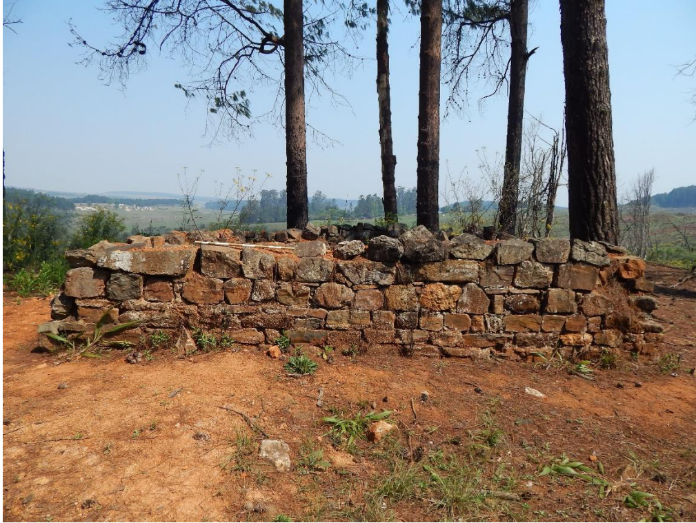
Fig. 7: The northern wall of the stone enclosure.
