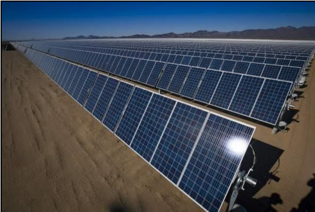
Photograph 1.1: Typical PV SEF facility
