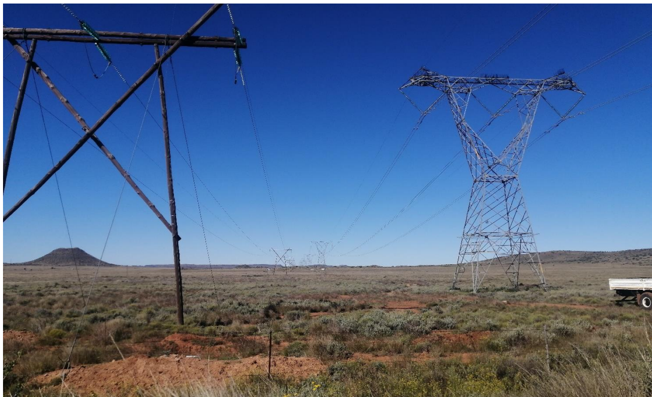
Figure 10: Electrical infrastructure that traverses the study area
