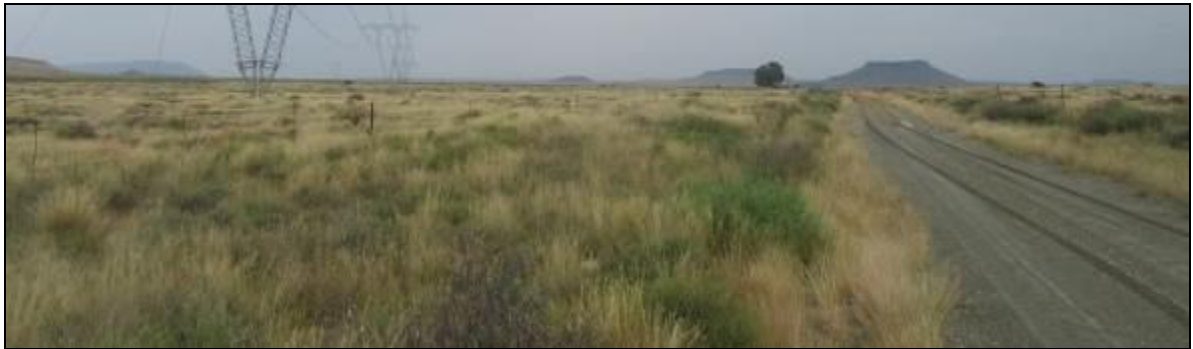
Photograph 3.4: Transmission line along the road between Tafelkop and Jakobsrus
