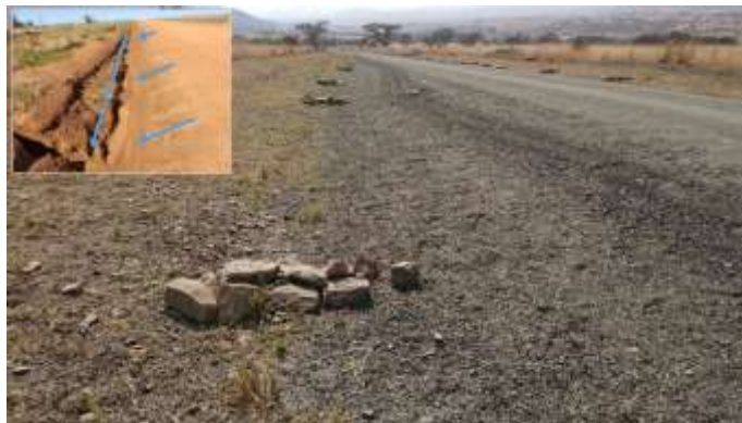
Figure 6-6 Example of road margin erosion prevention
