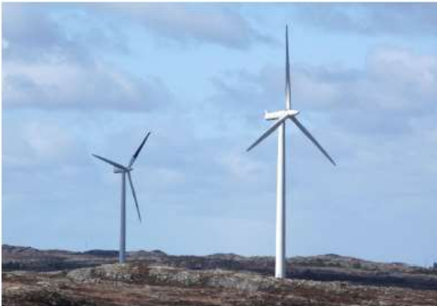
Figure 1: The black-blade set up on a cloudy day in Norway is shown left. The black-blade (far turbine) is little different to the shadow cast by the all-white blades in the foreground © Bjorn Iuell.
