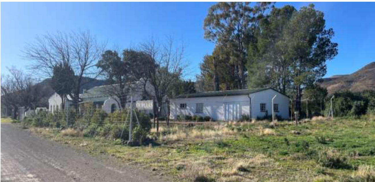
Figure 8: Example of homesteads located within the study area.
