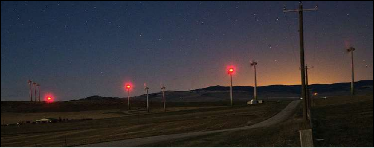
Figure 22: Aircraft warning lights fitted to the wind turbine hubs (Source: http://www.pinchercreekecho.com/2015/04/29/md-of-pincher-creek-takes-on-wind-turbine-lights )
