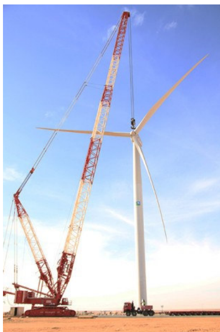
Figure 4-4: Crawler Crane used to assemble turbine (Liebherr, 2017)
