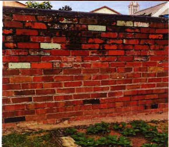
VIEW FROM PROPOSED SITE - LOOKING EAST
