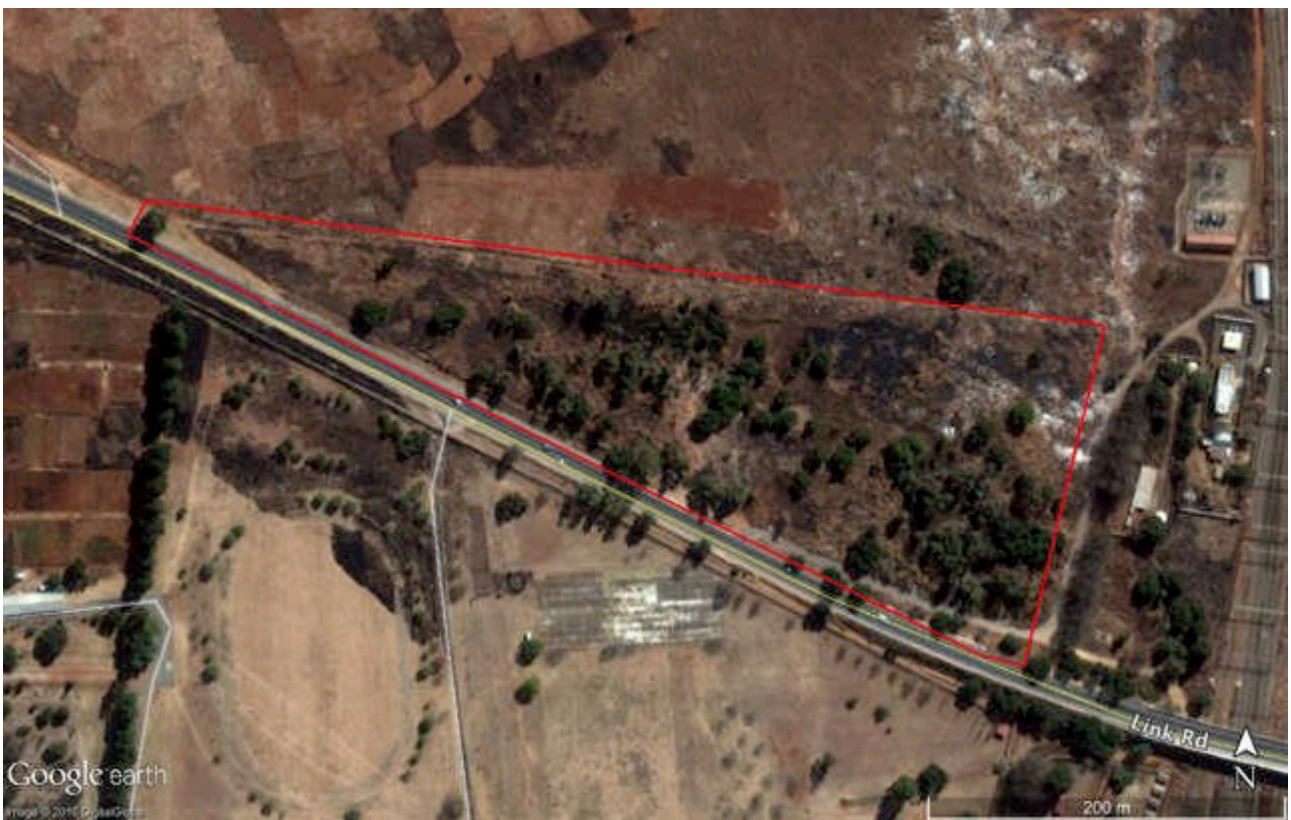
Figure 8 Google Earth image (2011/08/01) indicating increased dumping of rubble on the site and surrounding area as well as subsistence agriculture to the north
