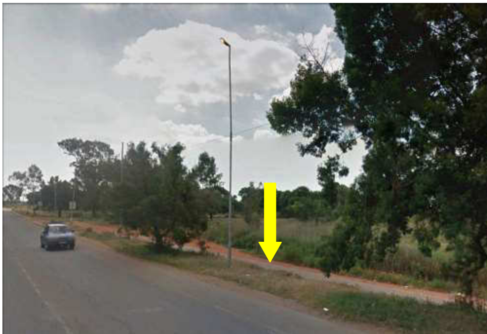
Transnet road next to Sam Molele Drive
